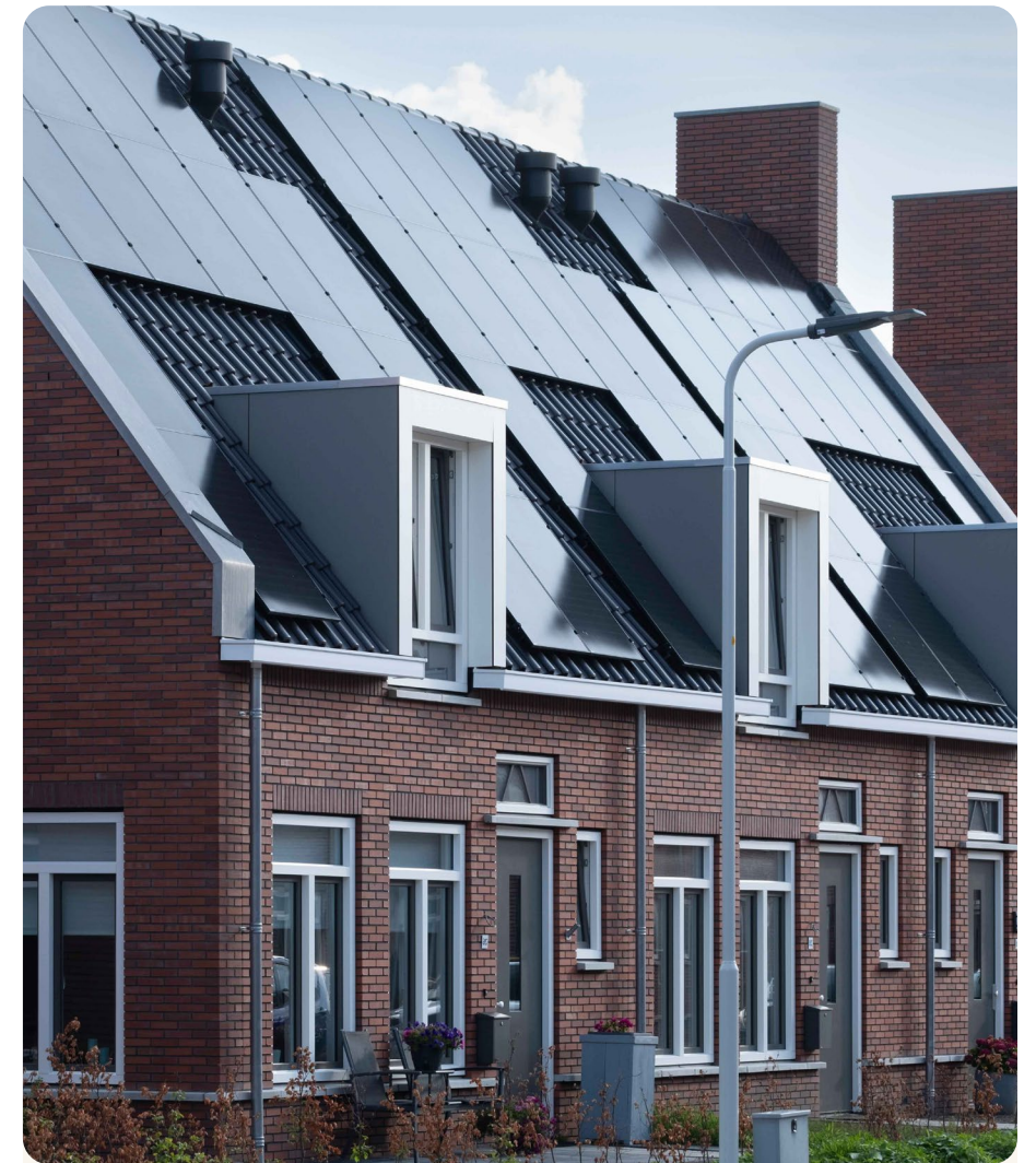
Solar panels on a social housing residence in the Netherlands
