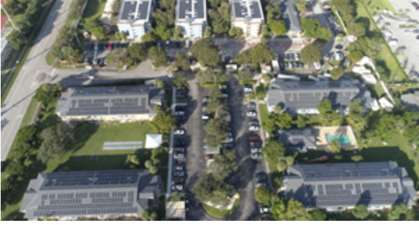
An aerial photo of the commercial solar system deployed by Urban Solar at Praxis of Deerfield Beach; the system is based on 1,798 Enphase IQ 7+™ microinverters
