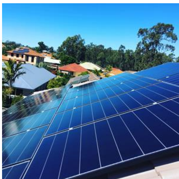
Enphase microinverters enable REA to install panel arrays across multiple roof areas and orientations to maximize solar power production.
